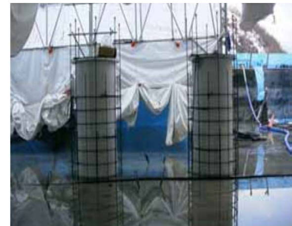
Embedding water level gauges
