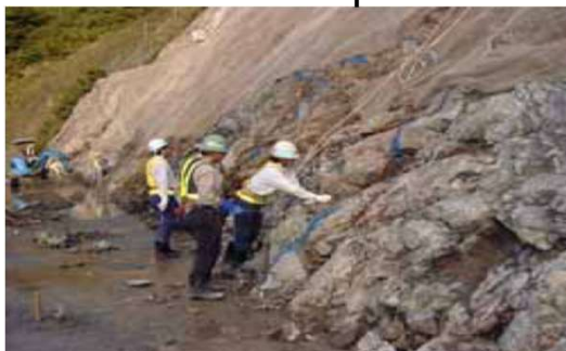
Rock foundation inspection before concrete placement
