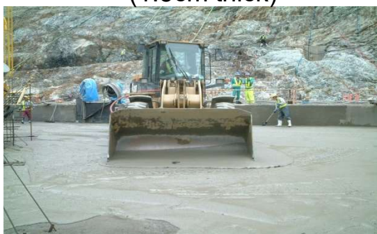
Mortar spreading, levelling (1.5cm thick)
