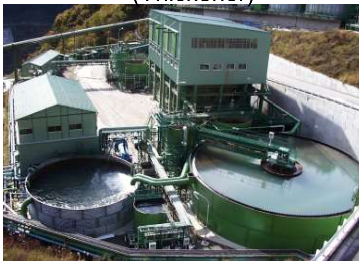
Turbid water treatment plant (Thickener)
