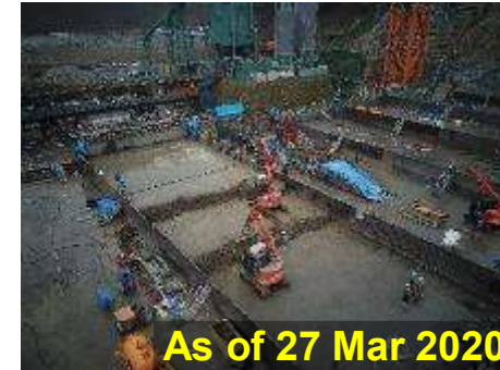
Concrete placement in progress
