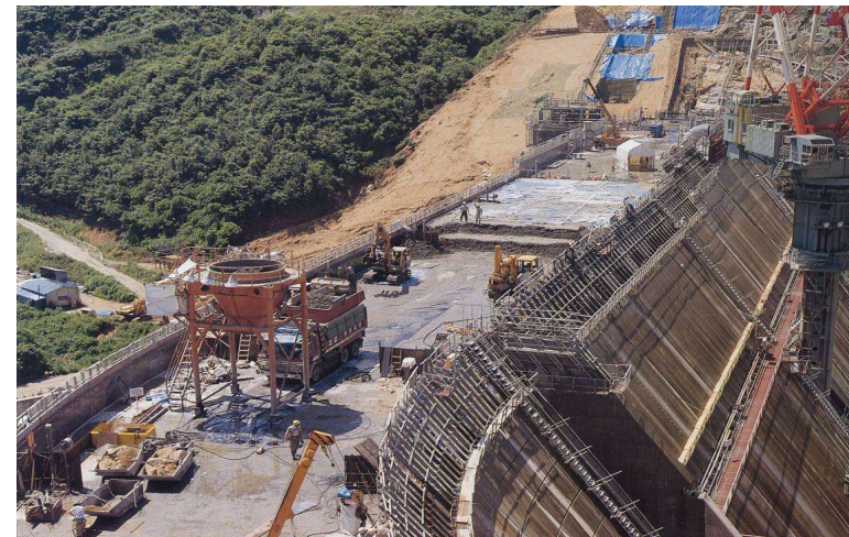
ELCM (Nunome Dam under construction)
