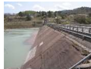
Minase Dam (Photo source: Dam listing)
