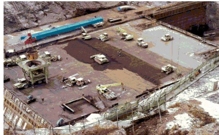
RCD Method (Tomisato Dam located in Ehime Pref.)
