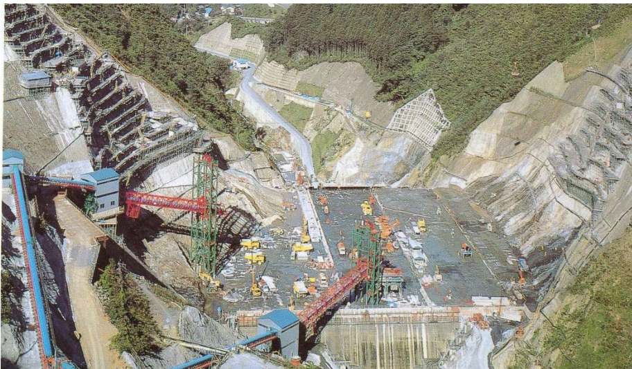
Construction of Urayama Dam (Dam height: 156m, Dam volume: 1.74 mil. m 3 )
