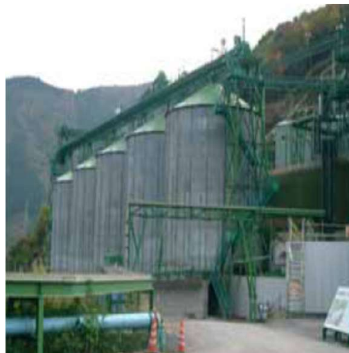
Storage bin for manufactured fine aggregate
