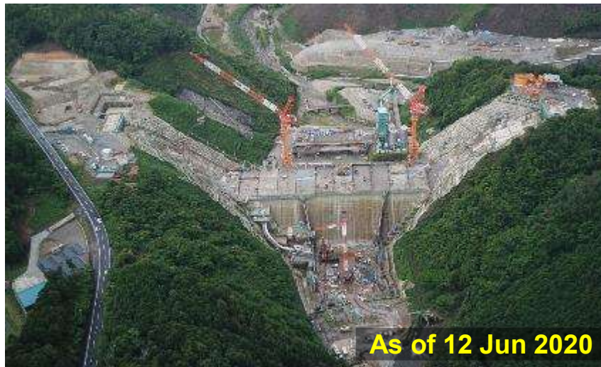
Bird-eye view of Kawakami Dam
