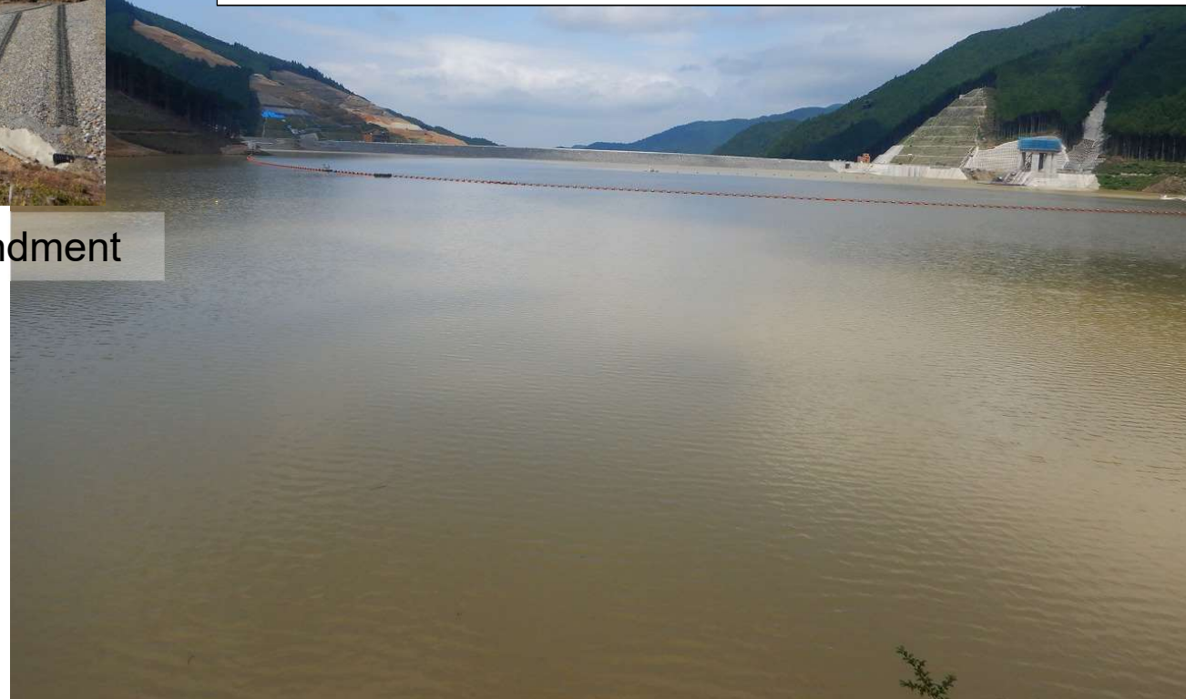
Full water reservoir (The dam body and the reservoir shot from the upstream)
