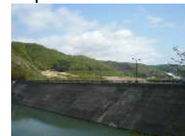
Ishibuchi Dam (Photo source: Dam listing)
