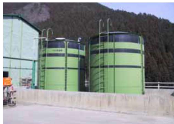
PAC storage tank
