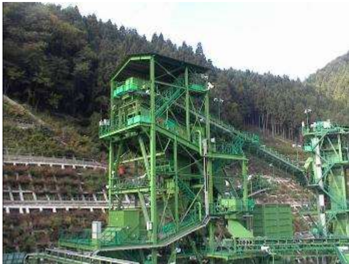
Sieving facility (Screen tower)
