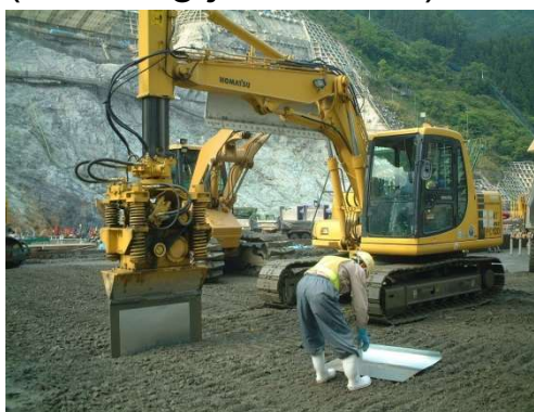
Joint creation (vibrating joint cutter)
